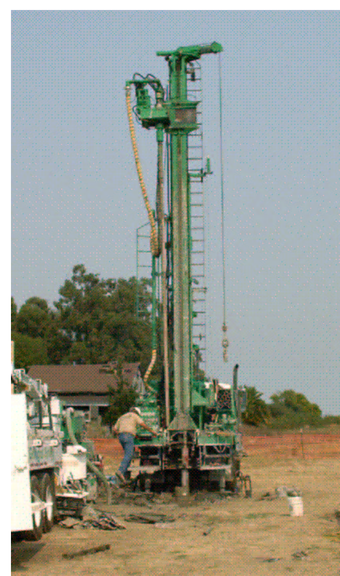
USGS Water Resources Division rig used to drill the borehole at St. Vincents.
