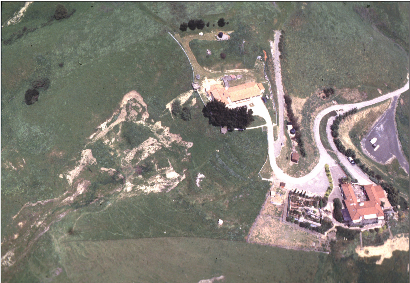
Figure 7. Slide behind houses with frontage along Eden Canyon Road. See map and figure 4 for location of photograph. Photograph taken April 22, 1998.
