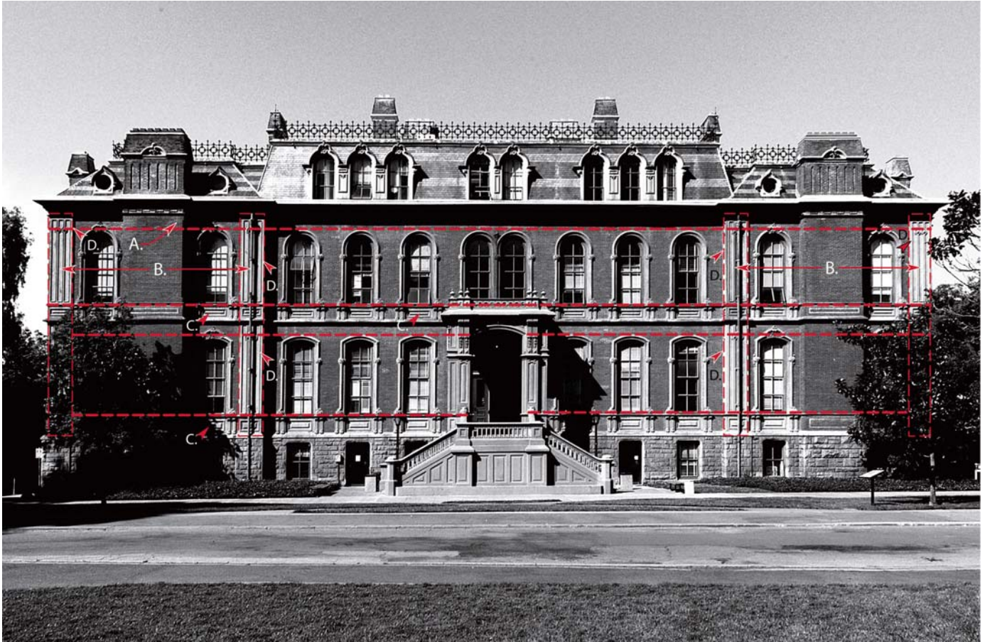
Figure 9. South Hall, 1873. Diagram of reinforcement in South Hall. A—bond iron courses through masonry; B—iron pilasters held in place by bond iron; C—the position of floor anchors in masonry; D—the position of internal iron girders.
