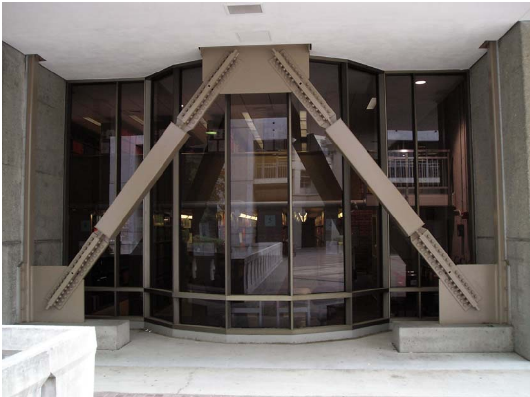
Figure 14. Hildebrand Hall: unbonded braces.
