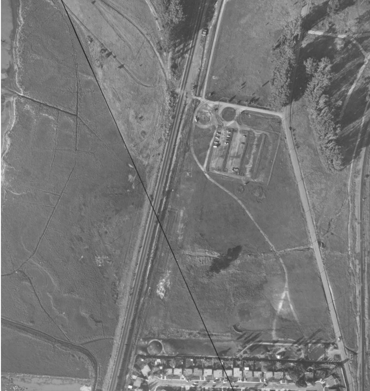
Figure 23. 1978 aerial photo of the Hayward fault as it passes through Parchester Village, offsets two pipelines and the Union Pacific railroad tracks, and then forms the linear scarp along the tidal marsh.
