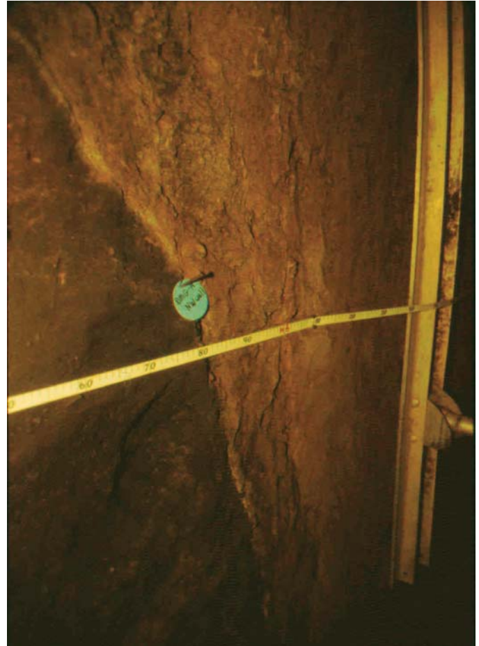
Figure 49. ( this and following page ) (A) Photograph of the Hayward fault exposure in a trench opened in 1987 on City of Fremont property (photo courtesy of San Jose Mercury News). The fault is a sharp boundary between fine-grained gray silt and light-colored sandy gravels.
