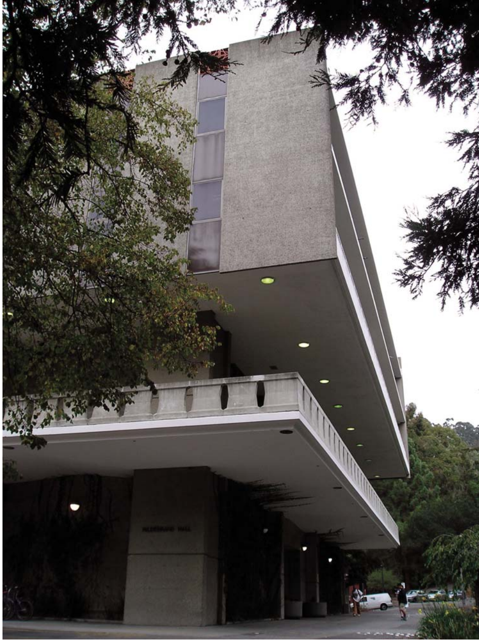
Figure 12. Hildebrand Hall seen from the southwest.
