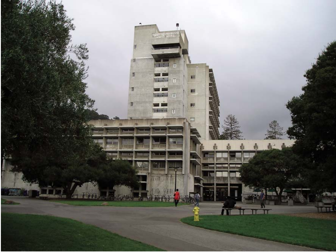
Figure 18. Wurster Hall, western façade.
