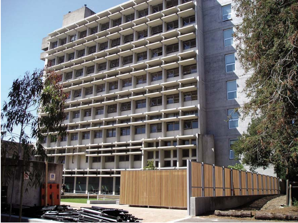
Figure 20. Wurster Hall Tower from the courtyard looking north.
